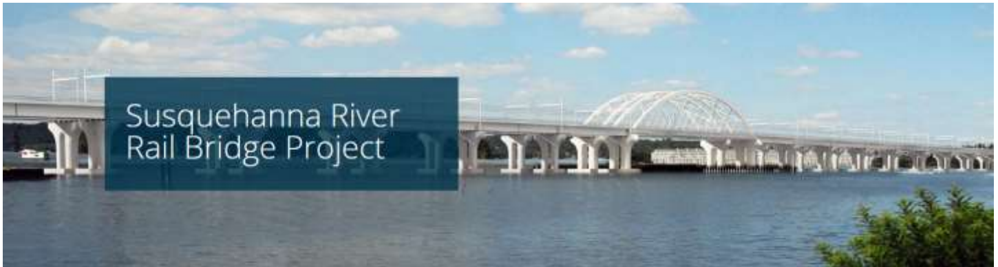
Amtrak's conceptual image of the 2 new bridges across the Susquehanna River from Havre de Grace to Perryville.
