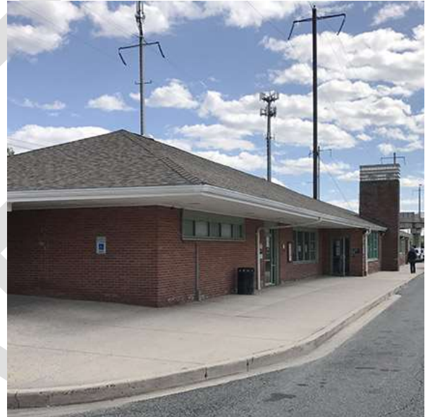
Built in 1943, the Amtrak/MARC passenger station in Aberdeen was designed by architect Lester C. Tichy.
