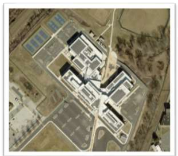
Aerial photo of the roof-top solar array, Havre de Grace Middle/High School, 2022
