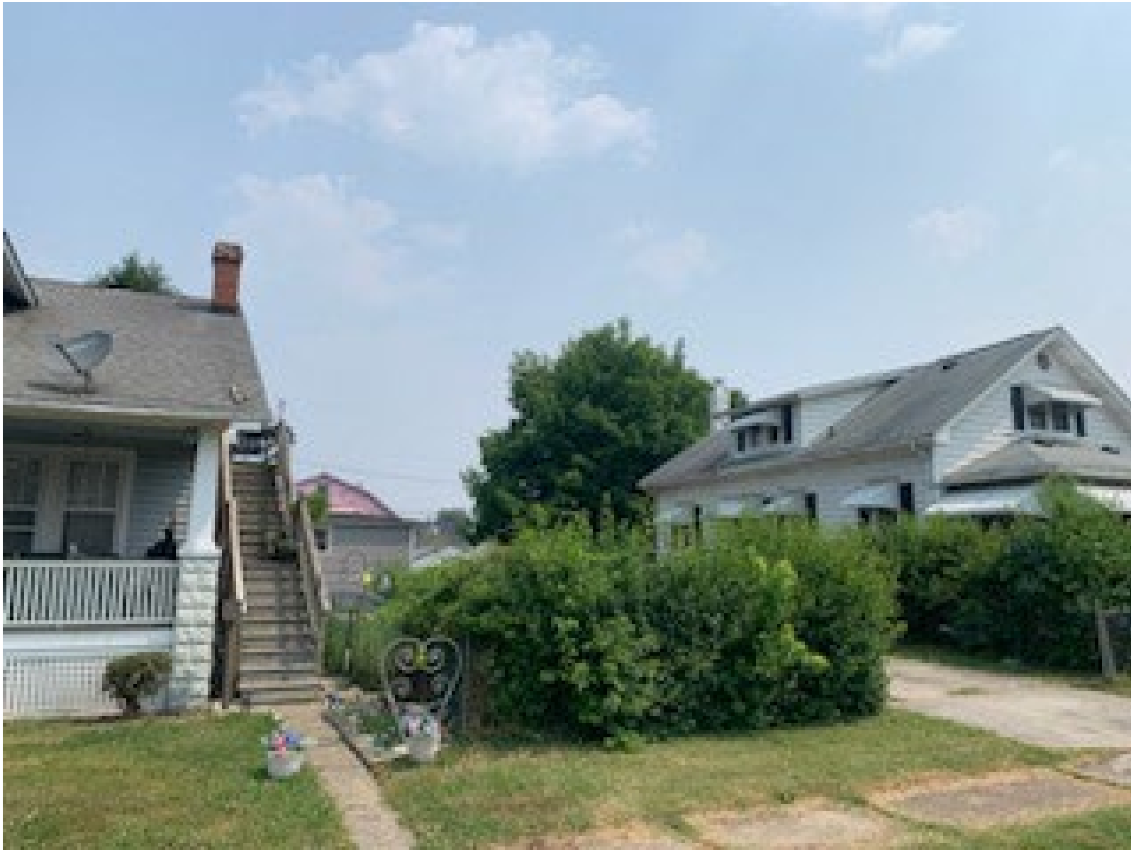
729 WARREN STREET- FACING NORTHEAST
