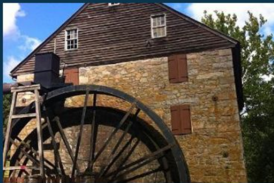
Rock Run Mill in Susquehanna State Park to the north
