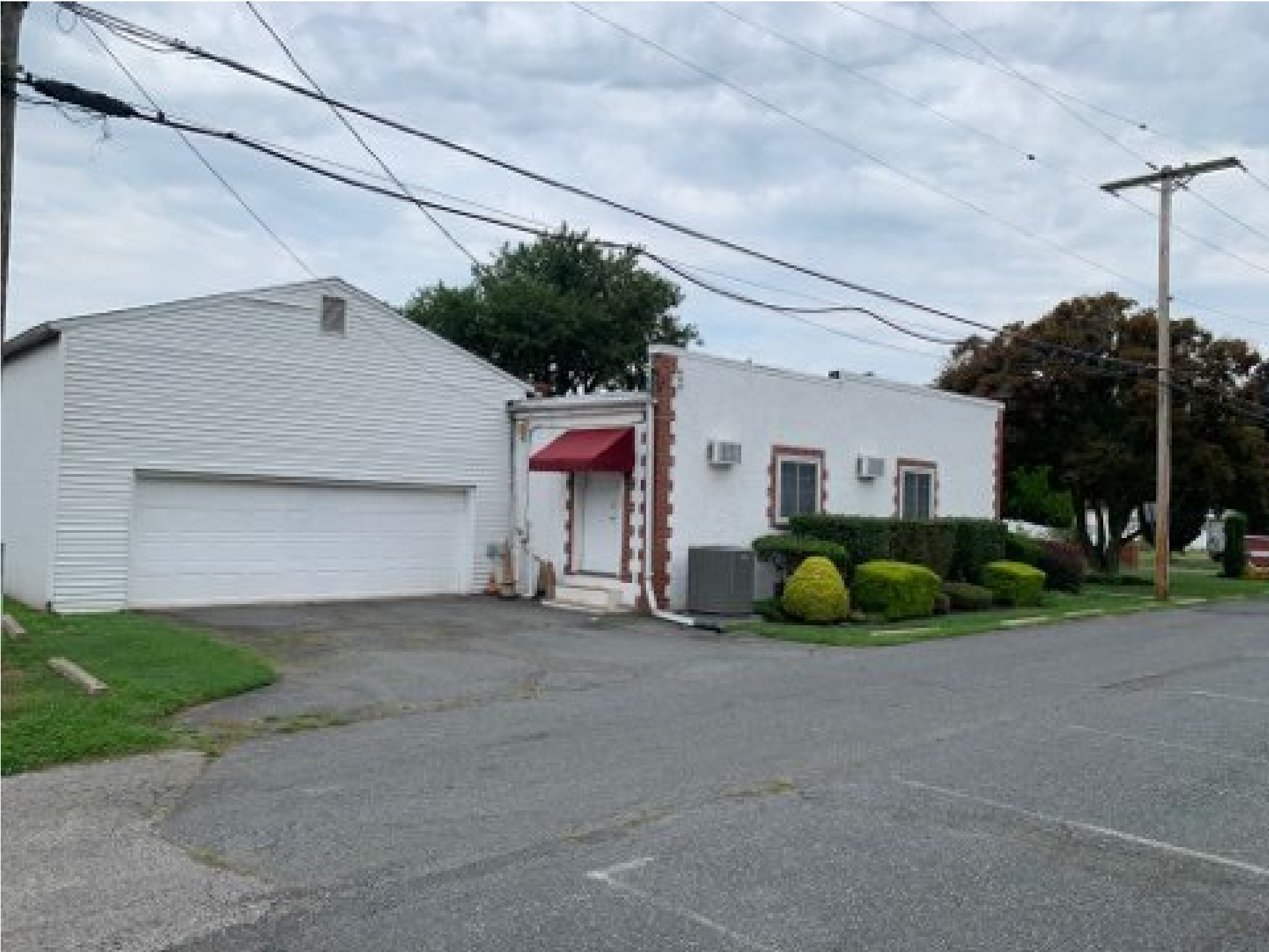
SOUTH FREEDOM LANE: FACING NORTH WEST-REAR GARAGE
