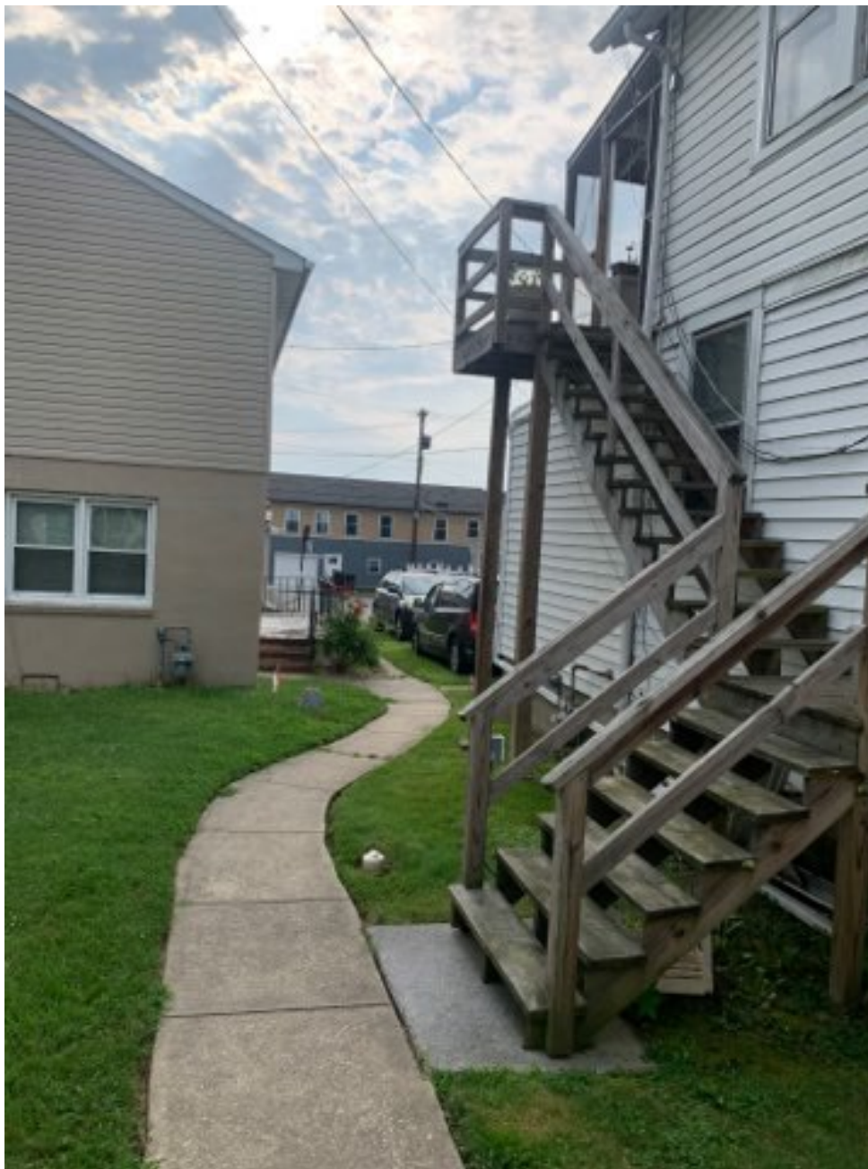
123-127 SOUTH WASHINGTON STREET: FACING EAST - SIDE CORRIDOR
