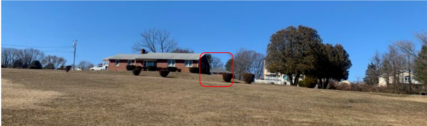
Facing North from Tydings Road
