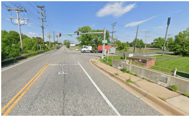
Figure 4a.- Looking north on Revolution Street at Old Bay Lane. Stancil Park Little League Fields are to the right.
