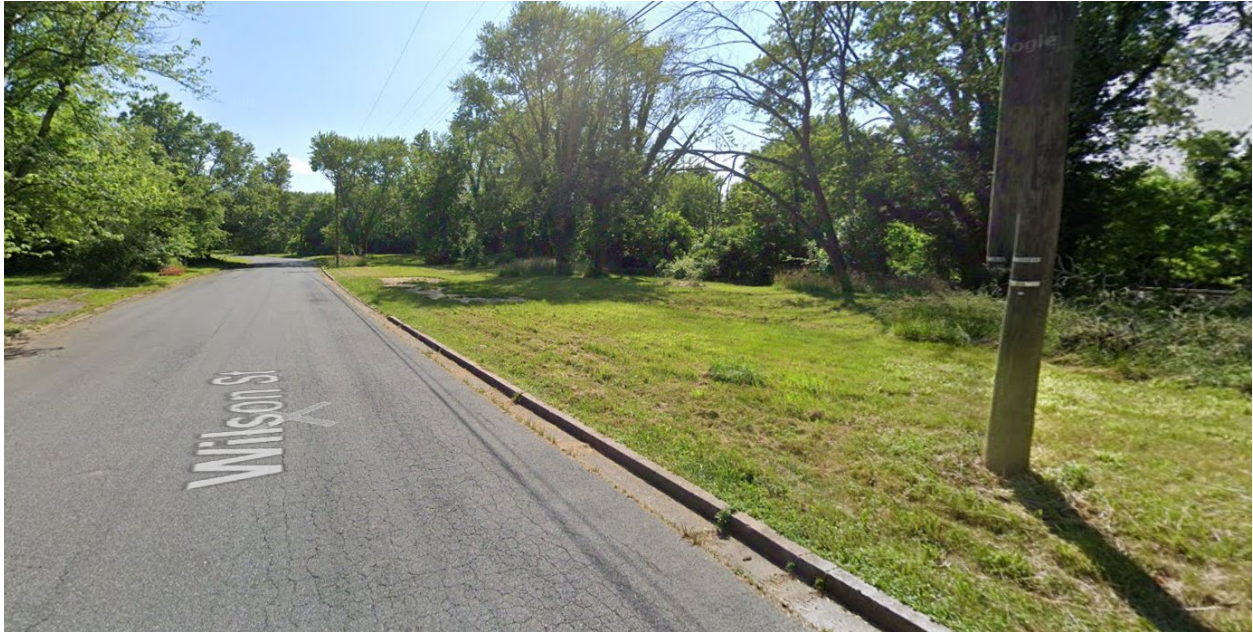
Figure 6. Wilson Street looking south. Norfolk Southern is behind the tree line to the right.
